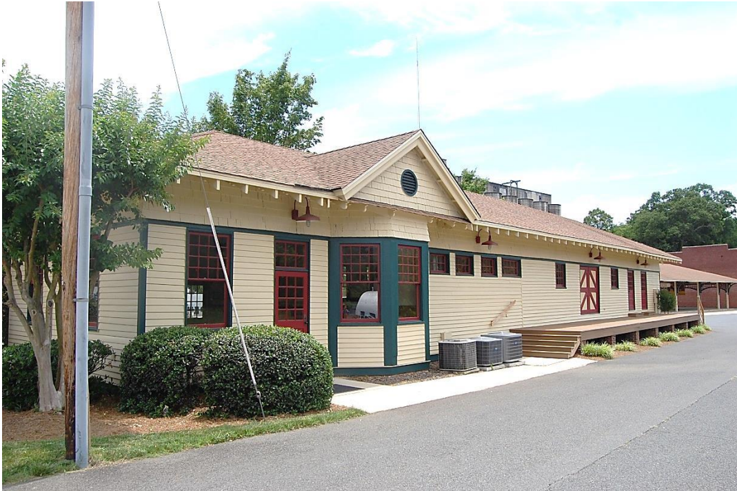
Winston-Salem Southbound Depot, West (Trackside) Elevation, Looking Southeast.
