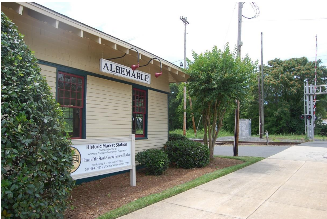
Winston-Salem Southbound Depot, North Elevation, Looking West From West Main Street.
