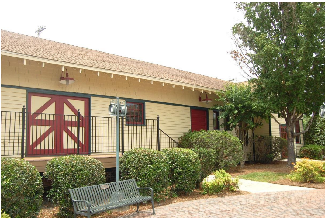
Winston-Salem Southbound Depot, East Elevation, Looking Northwest.
