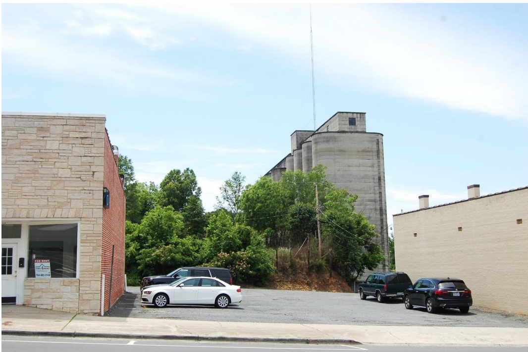
Albemarle Railroad and Industrial District, Southern Flour Mills Grain Elevators, Looking South From West Main Street.
