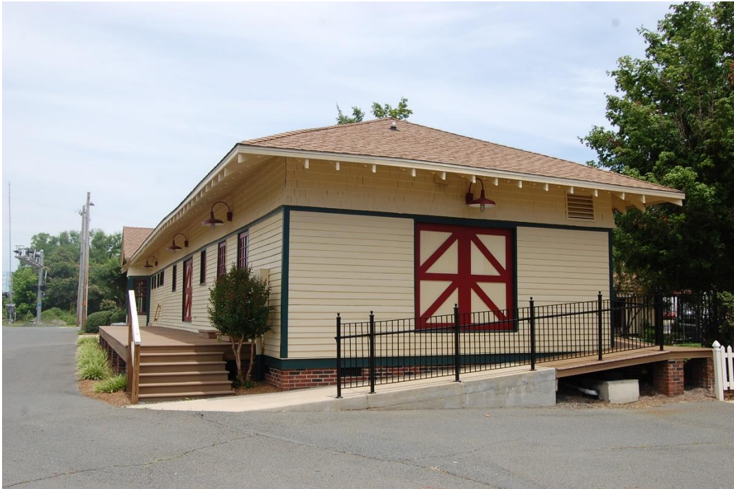
Winston-Salem Southbound Depot, South and West (Trackside) Elevations, Looking North.
