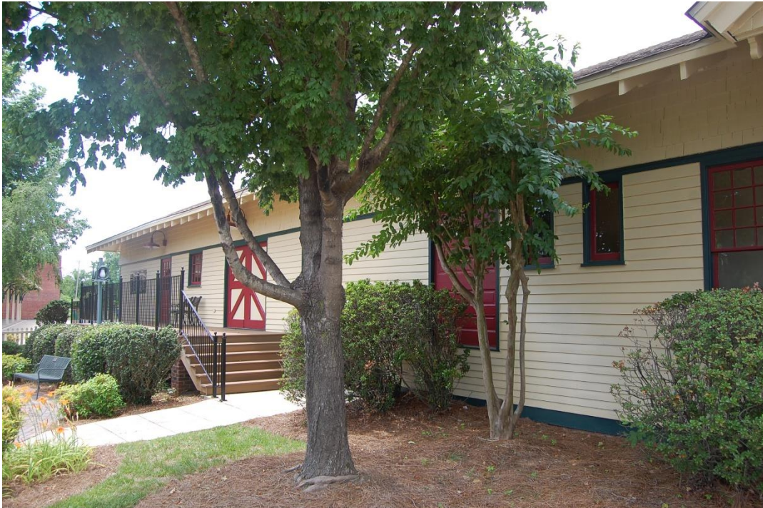
Winston-Salem Southbound Depot, East Elevation, Looking Southwest.
