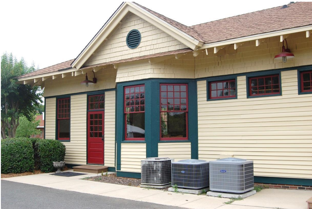
Winston-Salem Southbound Depot, West (Trackside) Elevation, Looking Northeast.
