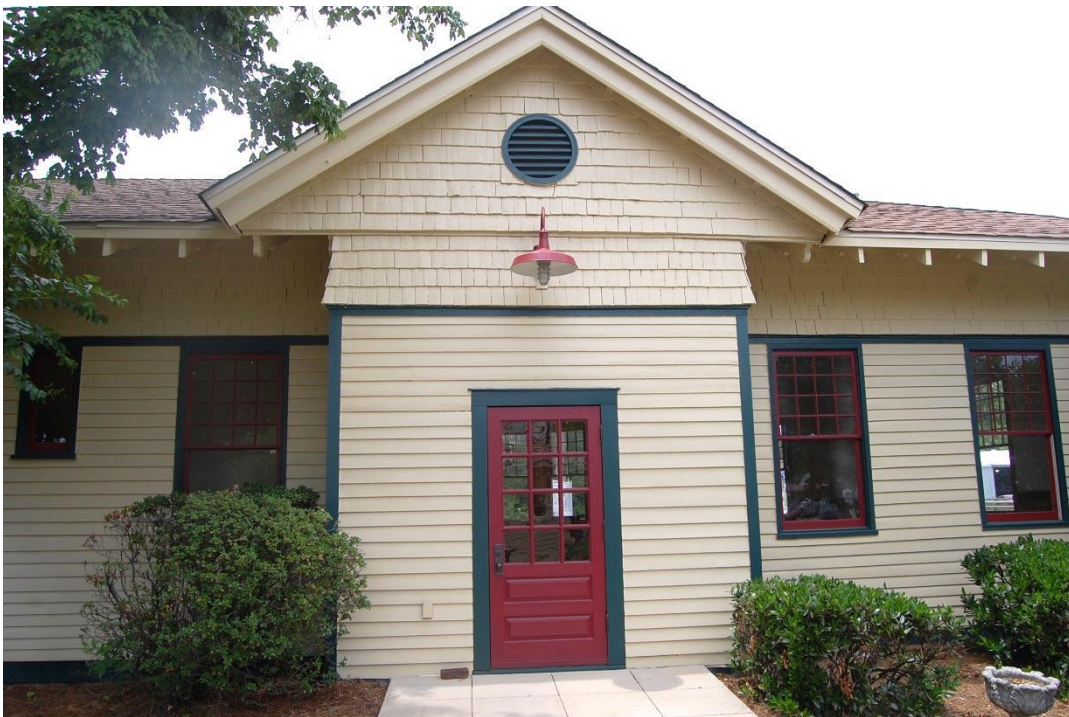
Winston-Salem Southbound Depot, East Elevation, Entrance, Looking West.
