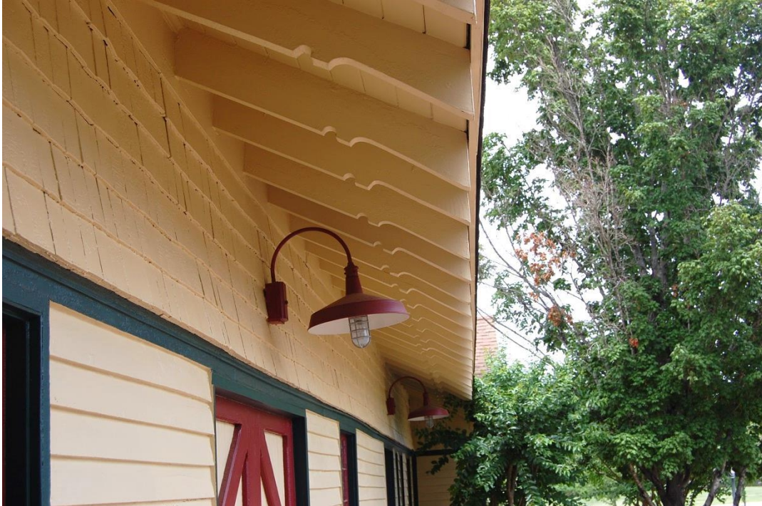
Winston-Salem Southbound Depot, East Elevation, Bracketed Eaves.
